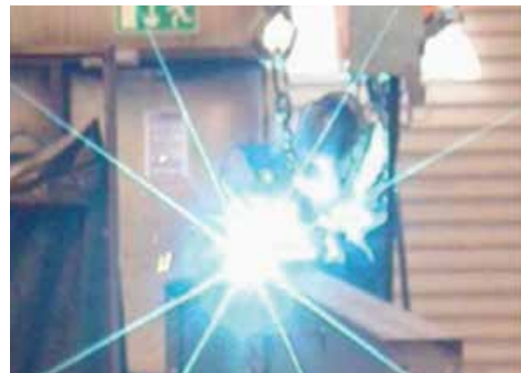
Now: Up to 70% reduction of harmful welding fume with the FOCUS.ARC welding process.
